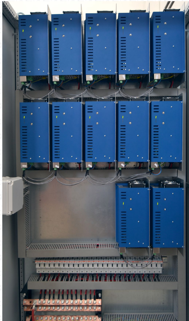
Figure 5 : Enclosure with integrated epic power modules
